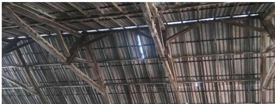
Picture 7 : Puducherry fire station with damaged roof
