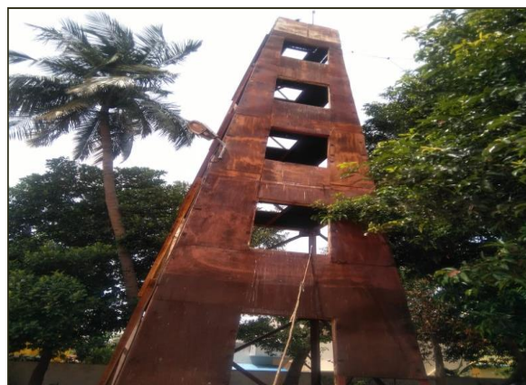
Picture 9 : Damaged tower without ladder
