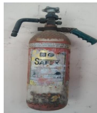
Picture 12 : Outdated fire extinguisher in Legislative Assembly
