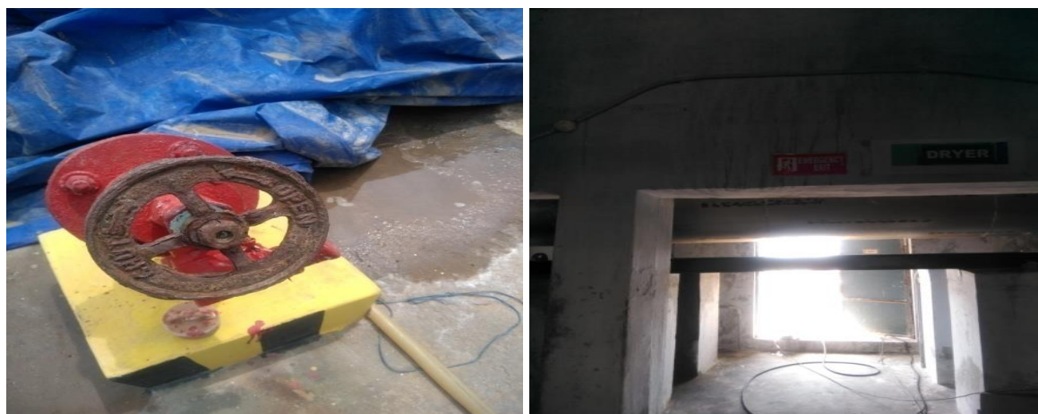
Pictures 10 and 11 : Inoperable Fire hydrant with rusted handle and fire exit obstructed with pipes (Vaigai Industries)
