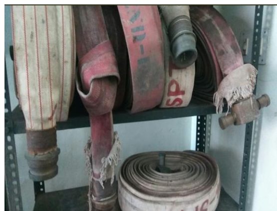
Pictures 5 and 6 : Worn out water hoses
