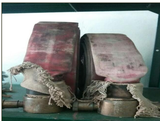
Pictures 5 and 6 : Worn out water hoses
